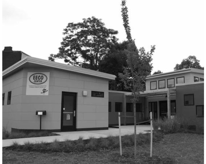
ABOVE: The EECO Center stands on the site of a former gas station at the intersection of East Liberty Boulevard and Larimer Avenue. Photo by Paula Martinac
